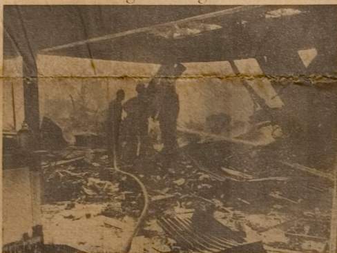
BUILDING RAZED —One of the several buildings which suffered severely in Sunday morning's raid over Honolulu was a large and old wooden structure at King and McCully streets. Here firefighters are shown amidst the bomb rubble trying to check the blaze which soon razed the building. (Advertiser Photo.)
