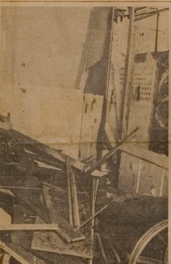
BOMB DAMAGE: The interior of the Paul Goo home at Lihua and Kuakini Sts., hit by a bomb.
